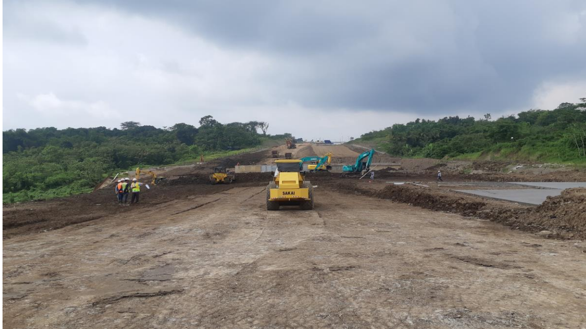
Soil Preparation Work
