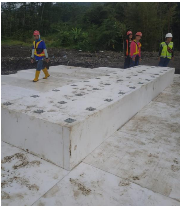
EPS Geofoam + GeoGripper Installation Work
