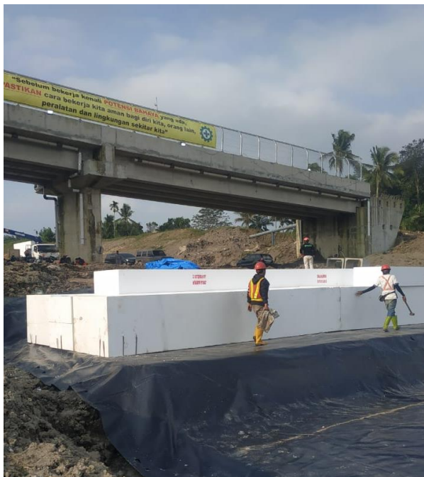
EPS Geofoam + GeoGripper Installation Work
