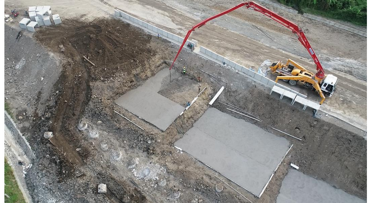
EPS Geofom Platform Work
