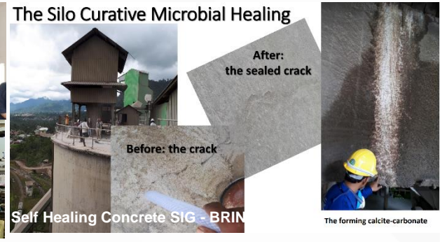
The Silo Curative Microbial Healing Self Healing Concrete SIG - BRIN The forming calcite-carbonate
