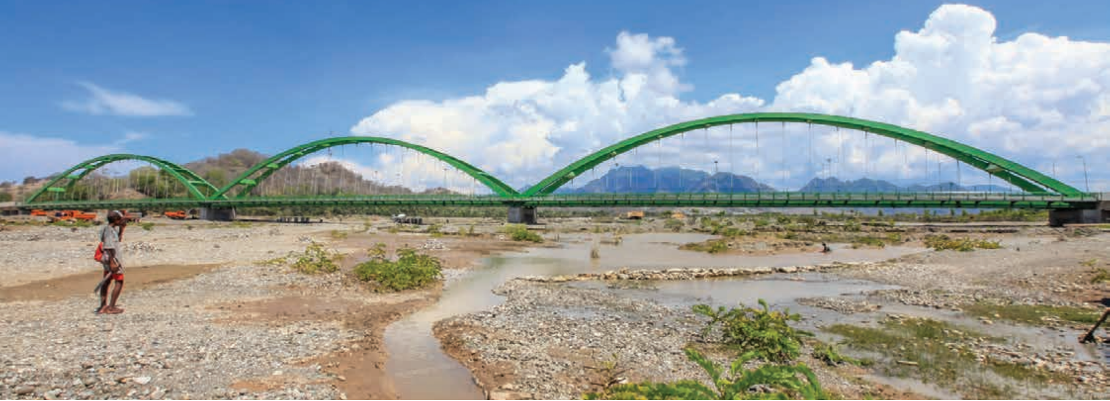
TONO BRIDGE - TIMOR LESTE
