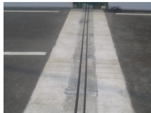
6 Ruas Toll Road
