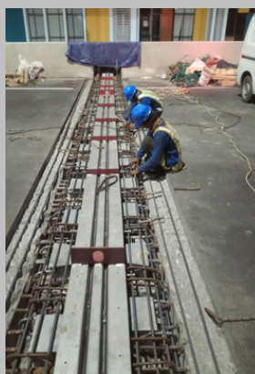
Modular Joint Installation on 6 Ruas Toll Road
