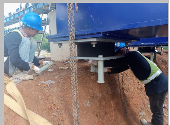
Lead Rubber Bearing (LRB) Installation on Bangkinang Pangkalan Bridge
