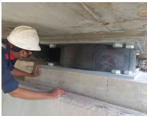
Aek Tano Ponggol Bridge
