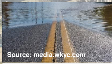
Vulnerable To Flooding
