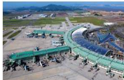
Tunnel, Airport, Dam
