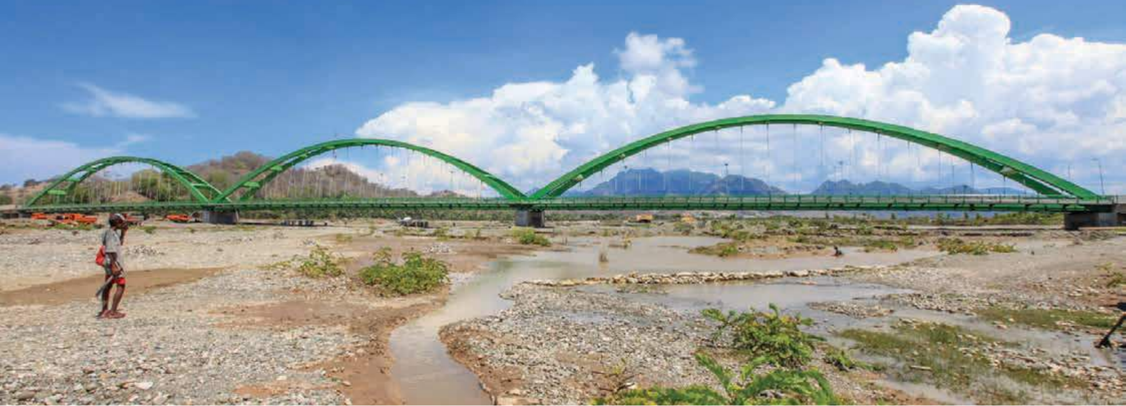
TONO BRIDGE - TIMOR LESTE
