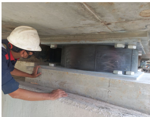
Aek Tano Ponggol Bridge
