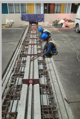
Modular Joint Installation on 6 Ruas Toll Road
