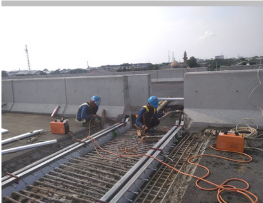
Strip Seal Joint Installation on Medan Binjai Toll Road
