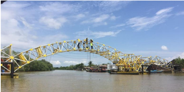
Floating Bridge ( Jembatan Apung ) technology in Cilacap, Central Java
