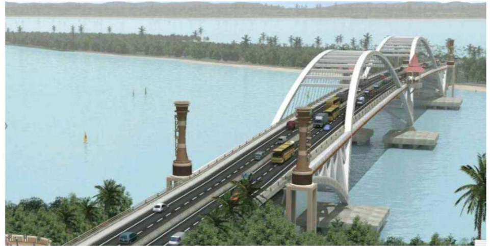
Holtekamp Bridge, Papua, Currently Under Construction
