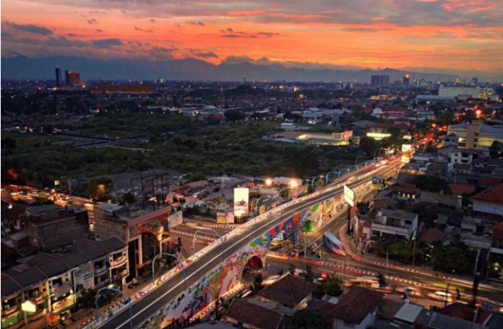
Utilization of Corrugated Steel in the construction of Overpass Antapani, West Java
