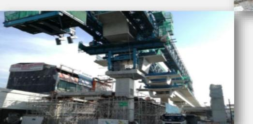
Girder elevation from road surface is 5 meters, which comply with the minimum requirements of vertical clearance according to public roads regulation
